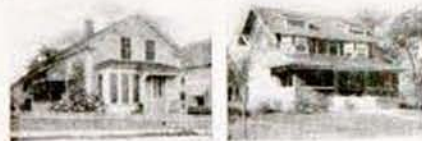
A No. 3015 IDEAL Boiler and 175 ft. of 38-in. AMERICAN Radiators, costing the owner $125, were used to heat this cottage. A No. 3-22 IDEAL Boiler and 400 ft. of 38-in. AMERICAN Radiators, costing the owner $215, were used to heat this cottage. At these prices the goods can be bought of any reputable, competent Fitter. This did not include cost of labor, pipe, valves, freight, etc., which installation is extra and varies according to climatic and other conditions.
