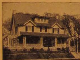
A No. 1-25-W IDEAL Boiler and 575 ft. of 38-in. AMERICAN Radiators, costing the owner $230, were used to heat this cottage. At this price the goods can be bought of any reputable, competent Fitter. This did not include cost of labor, pipe, valves, freight, etc., which are extra, and vary according to climatic and other conditions.
