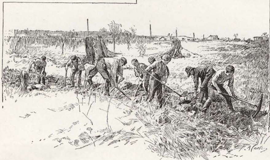
Digging a Ditch.
