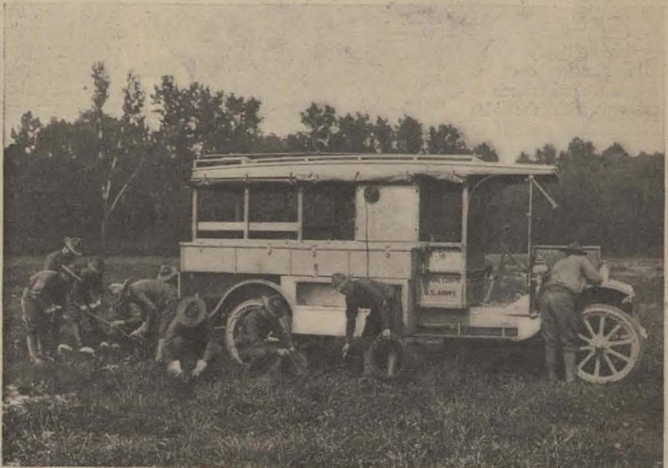
A DETACHMENT OF THE UNITED STATES ARMY SIGNAL CORPS LAYING A FIELD TELEGRAPH-WIRE DURING MANEUVERS
