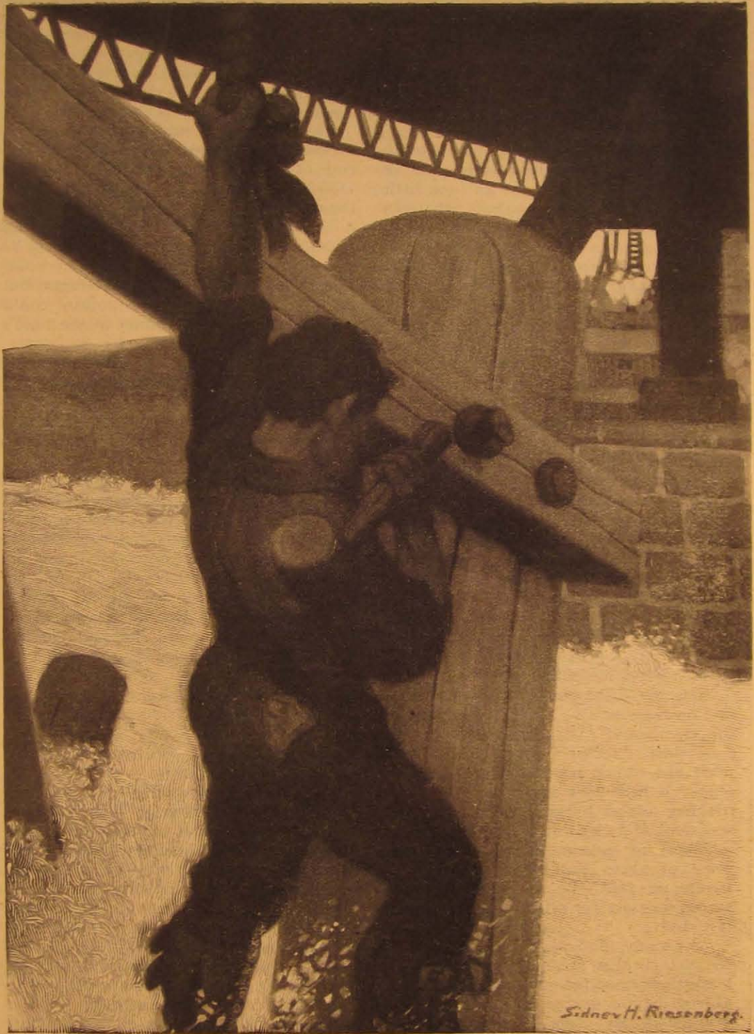
"Hanging by one hand and swinging a ten-pound hammer with the other"
