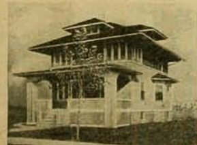
A No. 3-22 IDEAL Boiler and 600 ft. of 3/8-in. AMERICAN Radiators, costing the owner $255, were used to Hot-Water heat this cottage.
