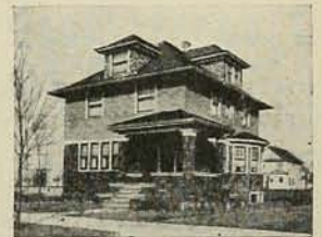
A No. 4121 IDEAL Boiler and 420 ft. of 38-in. AMERICAN Radiators, costing the owner $190, were used to Hot-Water heat this cottage.
