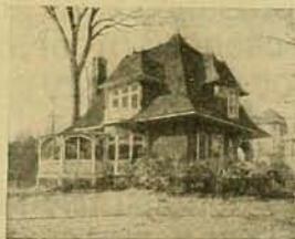
A No. C-241 IDEAL Boiler and 555 ft. of 38-in. AMERICAN Radiators, costing the owner $250, were used to heat this cottage.
