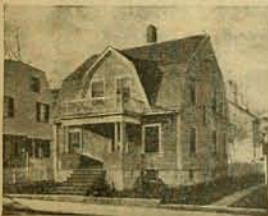
A No. 22 IDEAL Boiler and 240 ft. of 38-in. AMERICAN Radiators, costing the owner $115, were used to heat this cottage.
