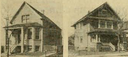
A No. 2118 IDEAL Boiler and 270 ft. of 38-in. AMERICAN Radiators, costing owner $135, were used to heat this cottage.
