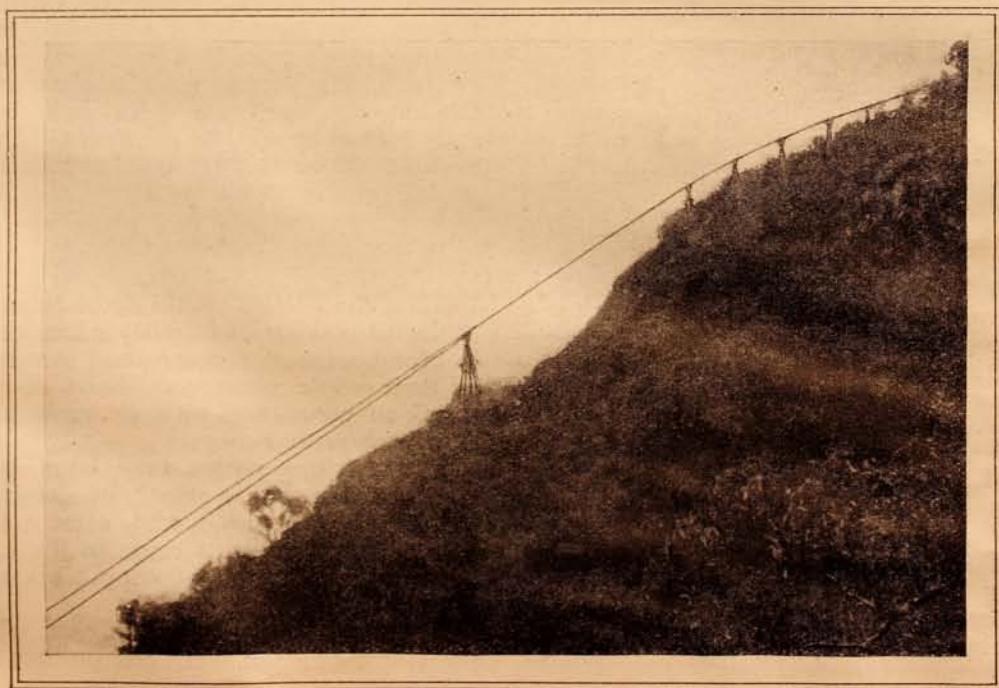
WHERE THE GERMAN EAST AFRICA "RAILWAY" BEGINS A DROP OF 6,600 FEET IN FIVE AND ONE-HALF MILES.
