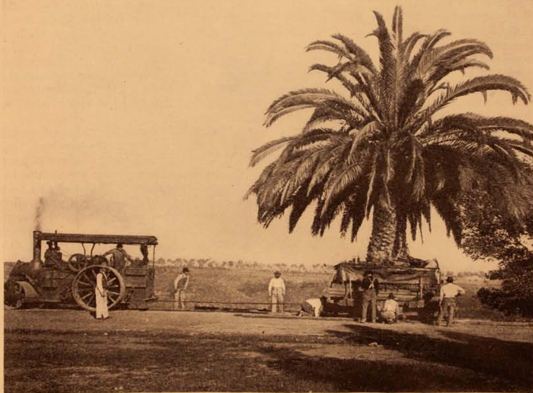
THE WORK OF TRANSFORMING BALBOA PARK, SAN DIEGO, CALIFORNIA, INTO AN EXPOSITION GROUND TO COMMEMORATE THE OPENING OF THE PANAMA CANAL OFFERS SOME PECULIAR METHODS OF TRANSPORTATION. HUNDREDS OF MASSIVE PALM-TREES, SOME WEIGHING FIFTEEN TONS, WERE TRANSPLANTED TO BEAUTIFY THE PARK. THEY WERE HAULED BY TRACTION ENGINES OVER ORDINARY ROLLERS.
