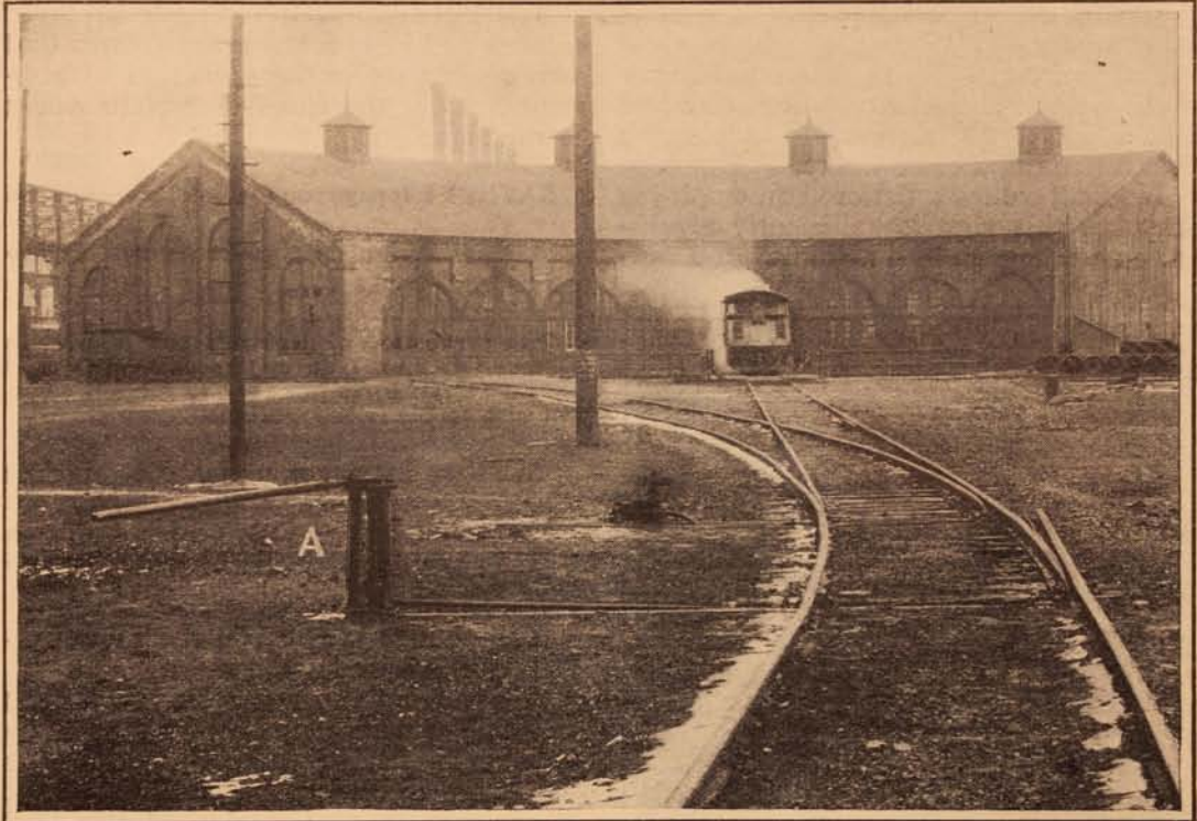
A.—ROUNDHOUSE DERAILING SWITCH. BEFORE REACHING THIS SWITCH AN ENGINE MUST STOP AND FIREMAN MUST HOLD THE SWITCH CLOSED FOR ENGINE TO PASS. WITHOUT THIS DEVICE AN ENGINE OR TRAIN NOT UNDER CONTROL MIGHT RUN INTO THE TURNTABLE PIT.
